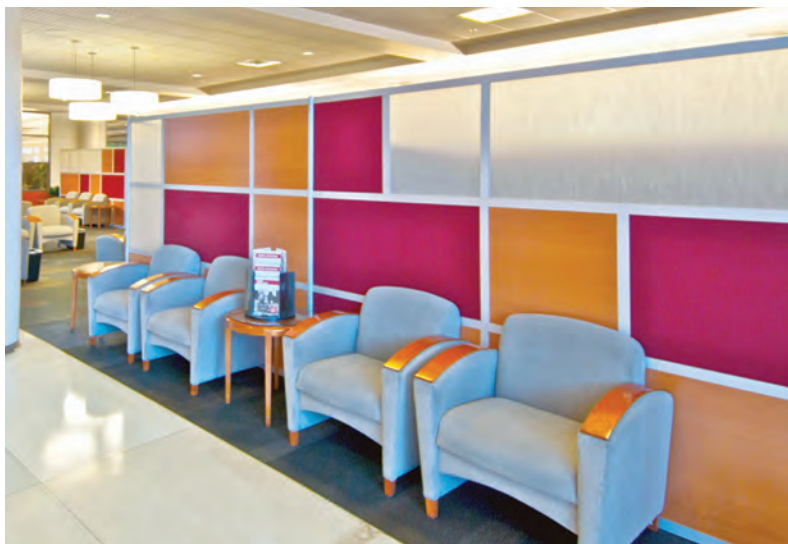
[Bottom Left] 20' wide custom wall with translucent colored and pearwood laminate panels
